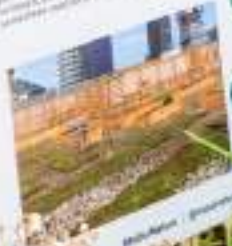
Printworks Green Roof
